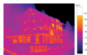
Thermal image with ScaleAssist
